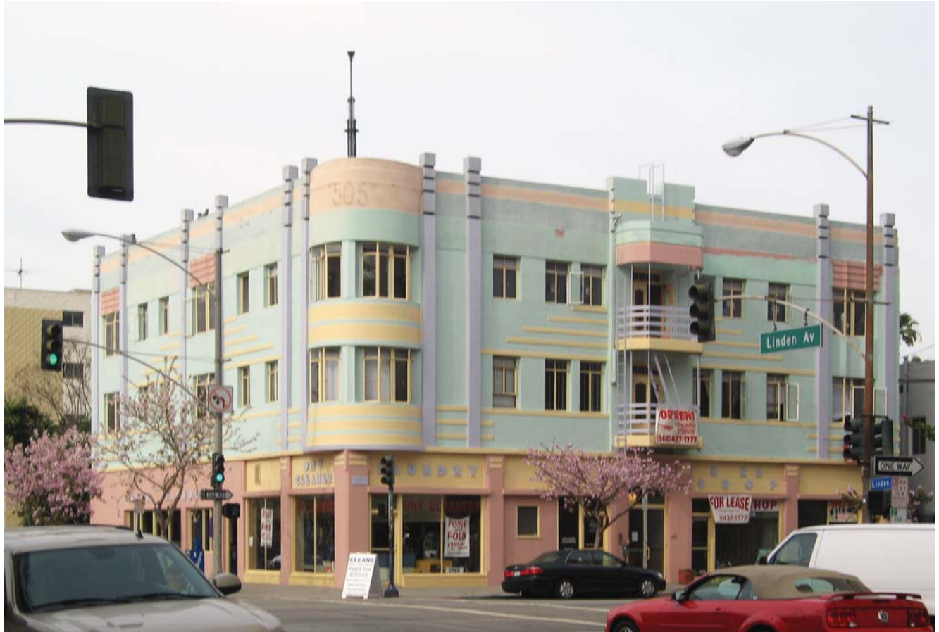
Metropolitan Apartments 501 East Broadway
