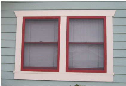
This compatible window screen is sized to the window and has a narrow wood frame painted to match the building's trim.
